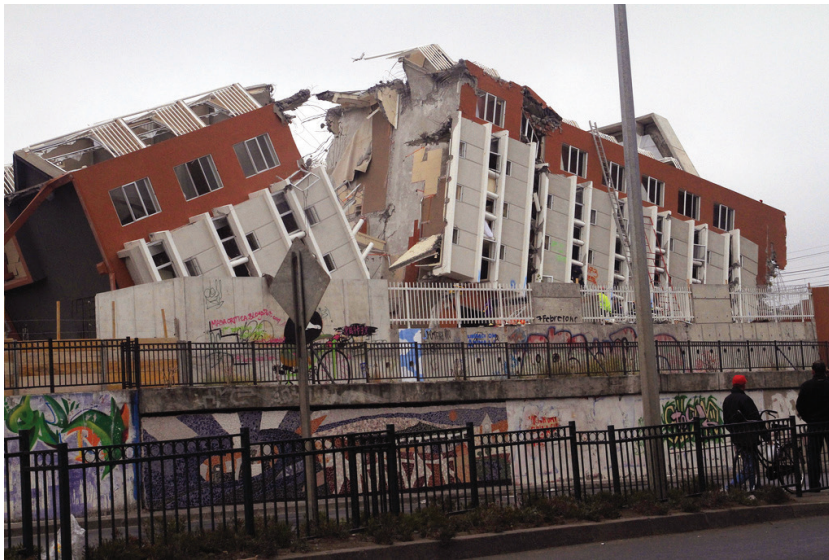
Collapsed building in Concepción, Chile, after a very large earthquake happened in February, 2010
